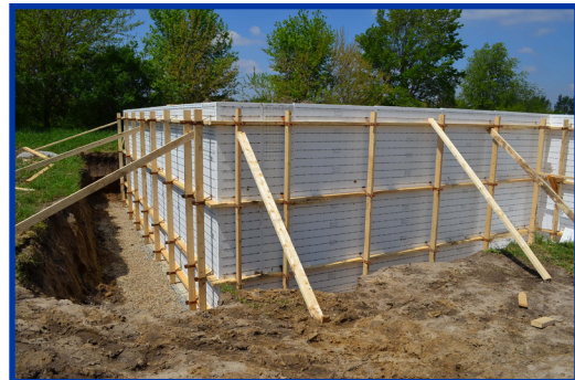
Image 2: Bracing on Exterior
