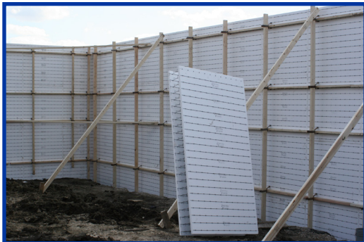
Image 1: Bracing on Interior
